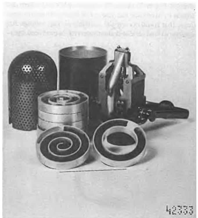
FIG. 10. Unidirectional ribbon microphone (1932).
