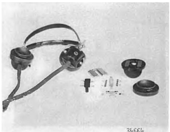
FIG. 7. High fidelity ribbon telephone receiver (1932).
