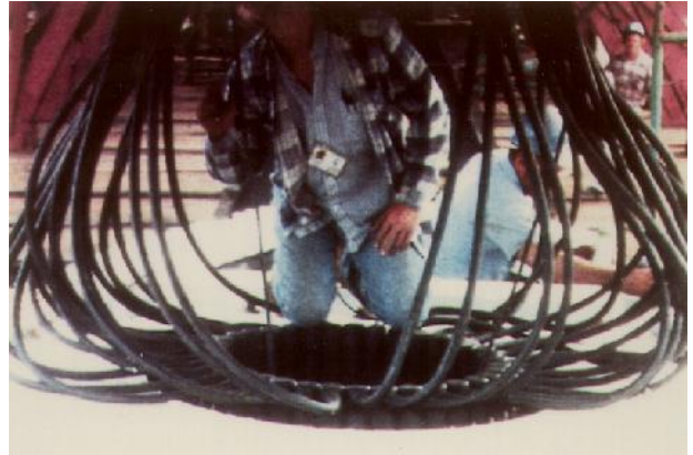
Photograph of Massa Stave Cables Being Installed on a Ship
